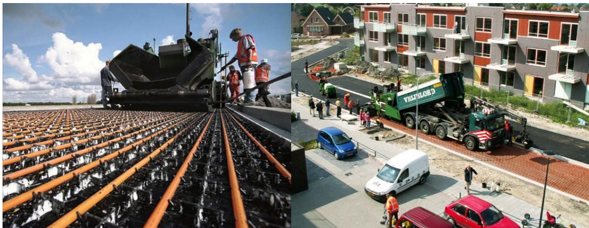
Figure 6: The use of pipework to extract heat from road surfaces for energy generation using aquifer heat exchangers in the Netherlands.
