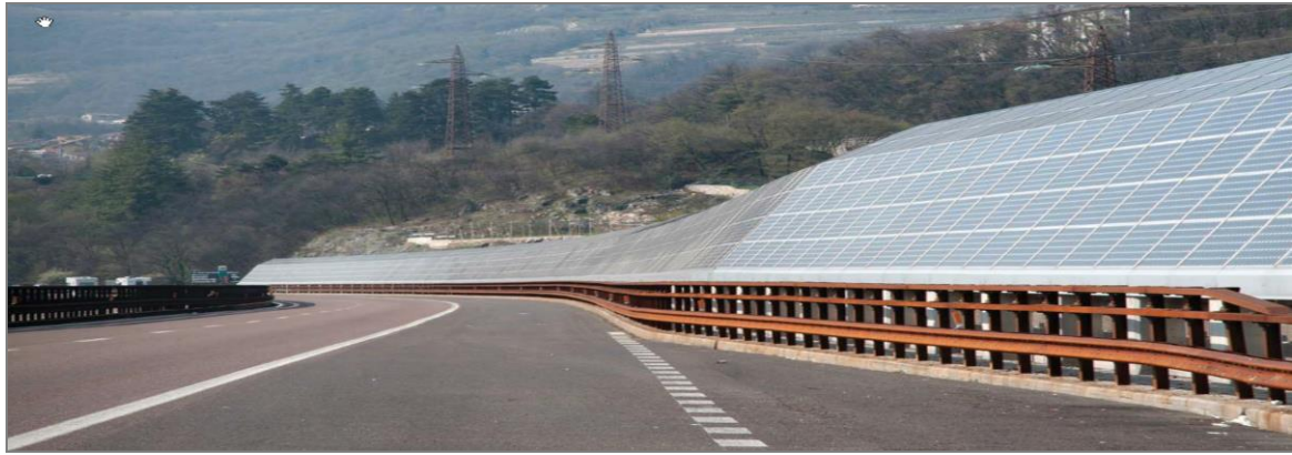
Figure 5: A photovoltaic noise barrier installed along the A22 Autostrada at Brennero in Italy.
