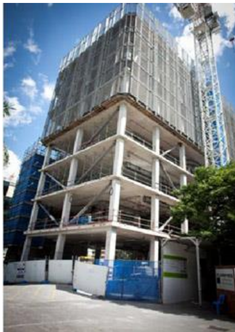
Figure 6: Structural steel cross-bracing used in the QUT Science and Engineering Centre (Source: QUT)
