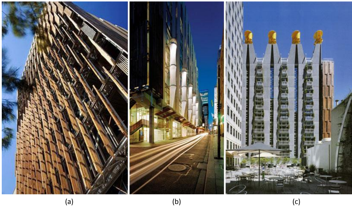
Figure 4: (a) Operable external shading (b) Evaporative Cooling System – Shower Towers, and (c) Variant Façade and Window Dimensioning. (Source: Melbourne City Council)
