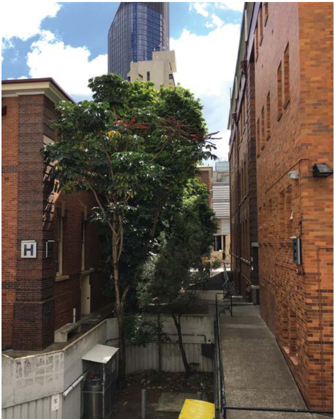
FIG 6.5.3.4: PHOTO OF CURRENT G - V BLOCK CONNECTION AT QUT GARDENS POINT.
