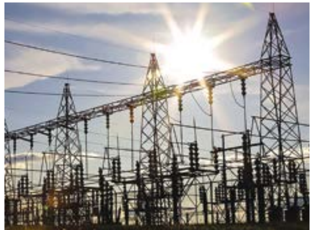
An innovation sprint helped Powerlink Queensland generate ideas to improve its asset security.
