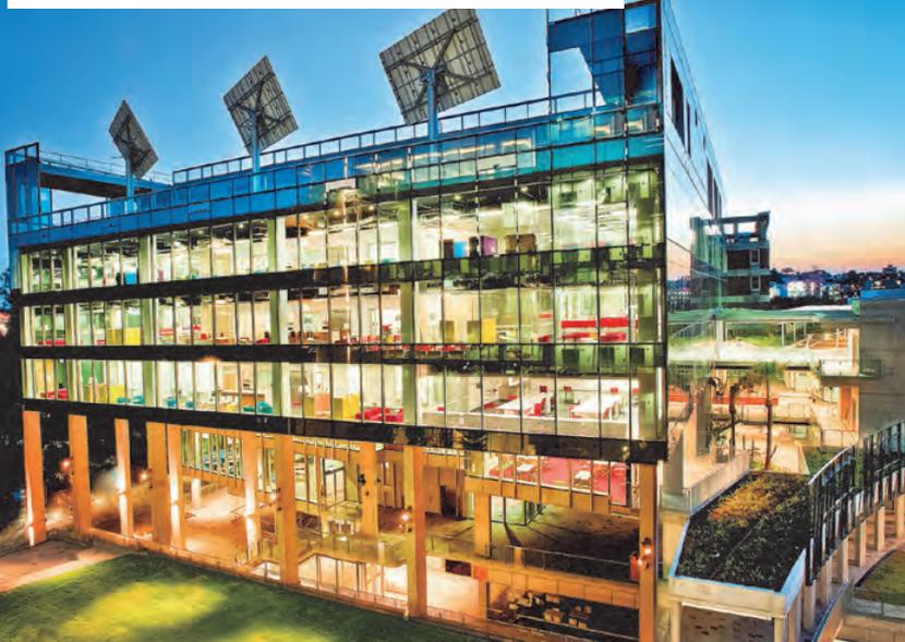
QUT's Science and Engineering Centre has a five-star Design Education VI certified rating from the Green Building Council of Australia. The building has a 200 kW solar PV array. Part of this array features three dual-axis trackers to align the modules throughout the day to achieve maximum power generation. When excess power is being generated, it can be fed into other buildings on campus.
