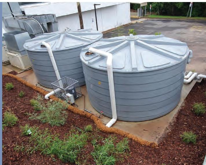
Two rainwater tanks at H Block, Kelvin Grove campus hold a total 68 000 litres (34 000 litres each tank).
